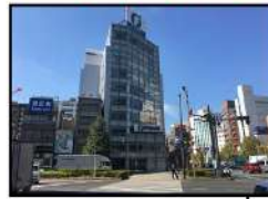
Distribution Hub Tokyo (Japan)
